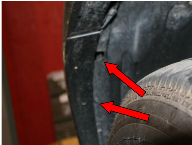
Figure 3 – Fenderwell fastener removal
